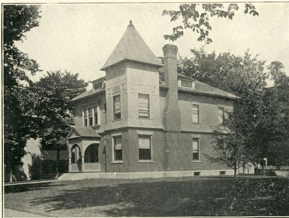
Hartford Library Building.
